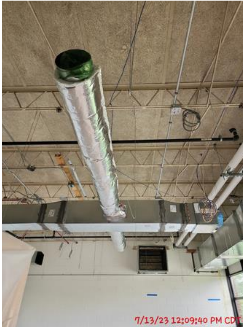
Mechanical Insulation
